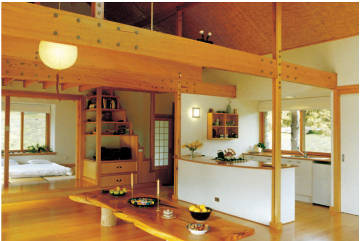
Post and beam structure
