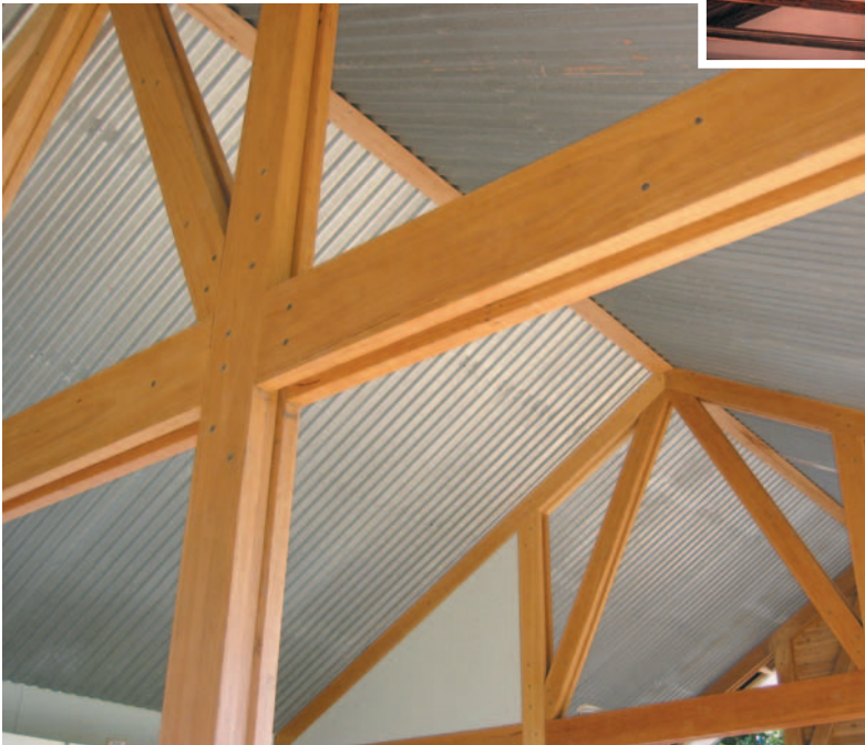
Expressed hardwood post and beam structure
