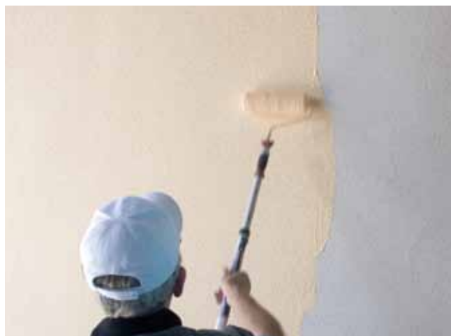
FIG 31: Applying Tinted Cemintel™ Top Coat
