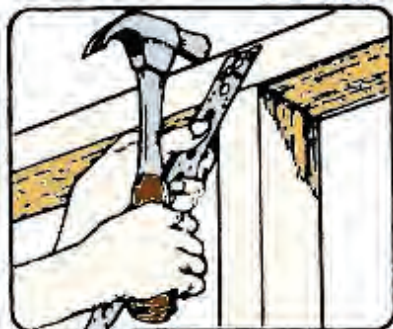
Hammer fixing to top plate
