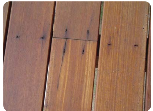
Incorrect use of non-galvanised ‘T’ head nails in decking.
