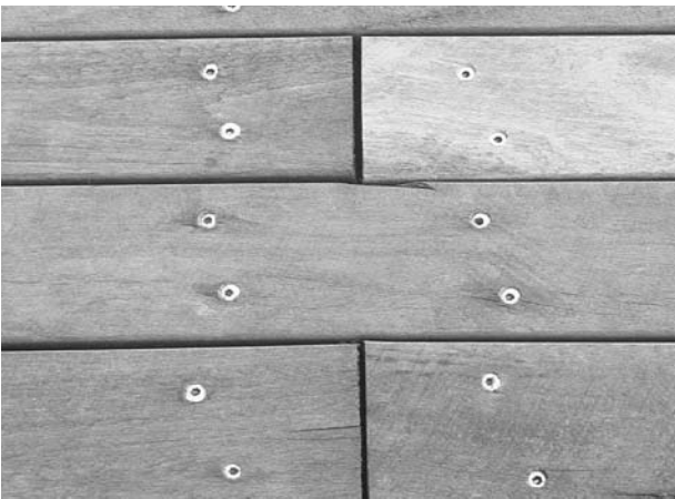
Joining over double joists
