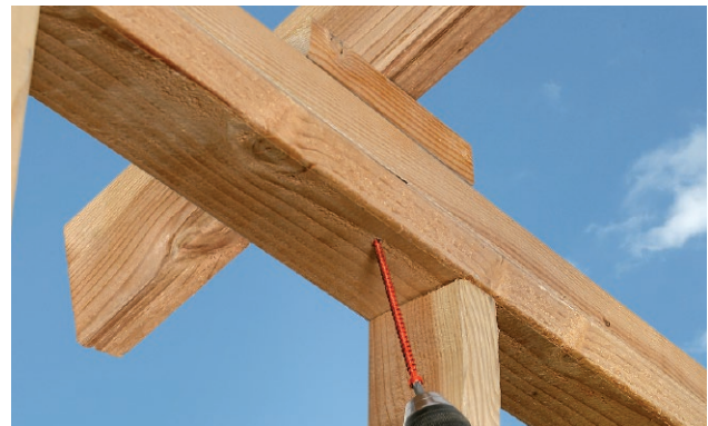
FIGURE 1 – Non-birdsmouth rafter with SDWC15600 installed with double top plates and rafter angle of 25°. Ceiling joist not shown for clarity. Connection is illustrated with 2-45 mm top plates.
