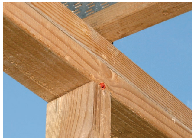
STEP 3 – Drive the SDWC until the head of the fastener is fully countersunk into the double top plate. Verify that the entire shank of the fastener is installed into a timber member.
