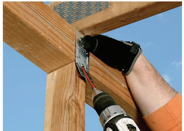
STEP 2 – While continuing to drive the SDWC, “drop” the fastener head into the guide channel to ensure optimal installation angle of 22°. The installation angle range is 10°-30° (see illustration). Once the installation angle is established, the metal installation guide tool may be removed.
