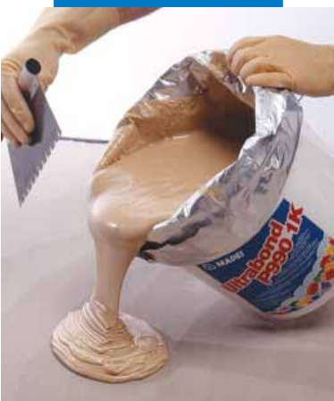
Pouring the adhesive on a screed
