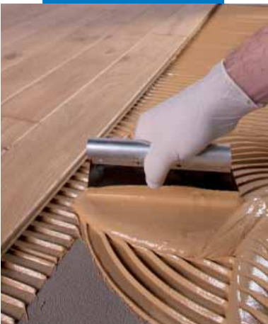
Spreading Ultrabond P990 1K
