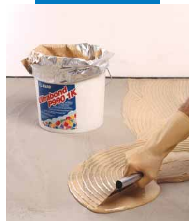
Spreading the adhesive
