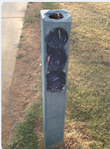
B: Reinstated – The damaged bollard is about 10 years old and is shown reinstated with the aid of a steel picket.
