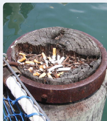
C: Deterioration at heart – Traditional steel banding to bollard ends does nothing to protect the post from weathering.
