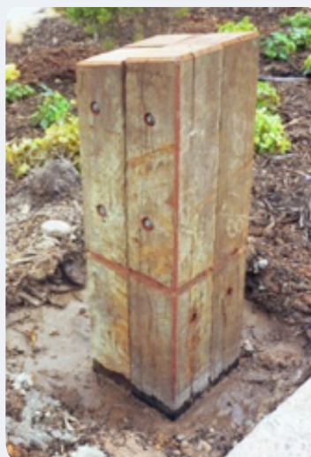
Figure 8.1: The illustrated composite bollards were built on the same project at different stages. The image A bollard has four spotted gum species members bolted together to gain a mass appearance.
