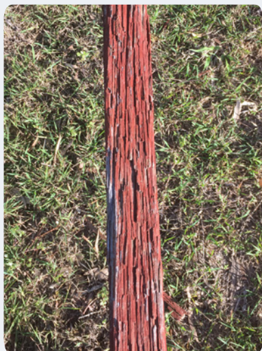
A: Top rail weathering – Some degradation apparent in more than 30 years of weathering.
