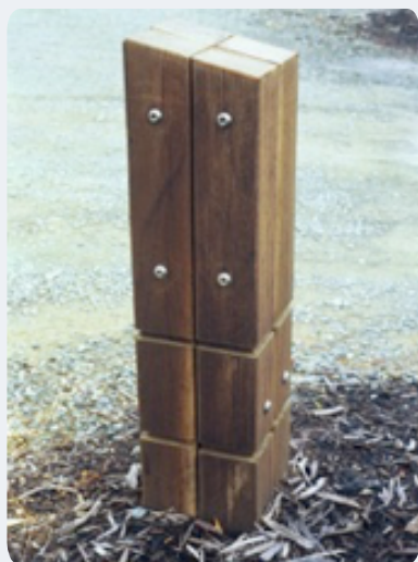
Figure 8.1: The illustrated composite bollards were built on the same project at different stages. The image A bollard has four spotted gum species members bolted together to gain a mass appearance.
