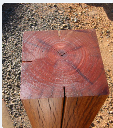
B: Controlled movement – Using a router to provide a groove over a sawn line controls surface splitting and avoid splinters.
