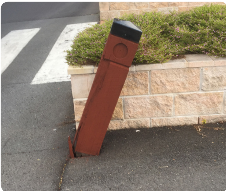
Figure 6.2: Providing a free-draining foundation for bollards limits the potential for moisture build-up and thus decay.
