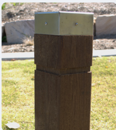
A: Over-fitted – Simple push-on end cap requires accurate symmetrical post cutting and ideally discrete fixing.
