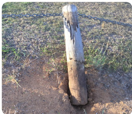
Figure 6.1: Bollards buried in ground should aim for 600 mm deep to avoid overturning.
