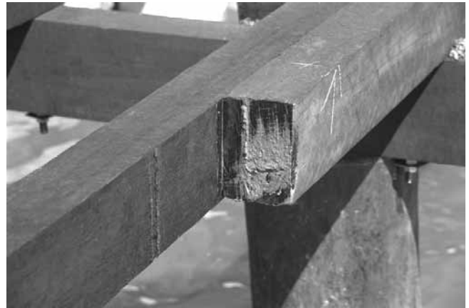
Fig 21 CN Emulsion on cut end
