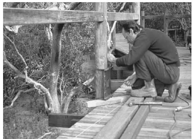
Fig 18 Round handrail post system - router jig
