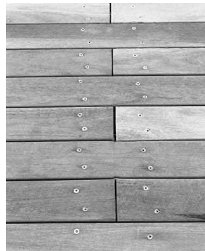
Fig 22 Staggering of plank joints in wide sections of decks is facilitated by paired joists
