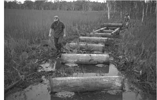
Fig 37 Bedlog installation on poor ground
