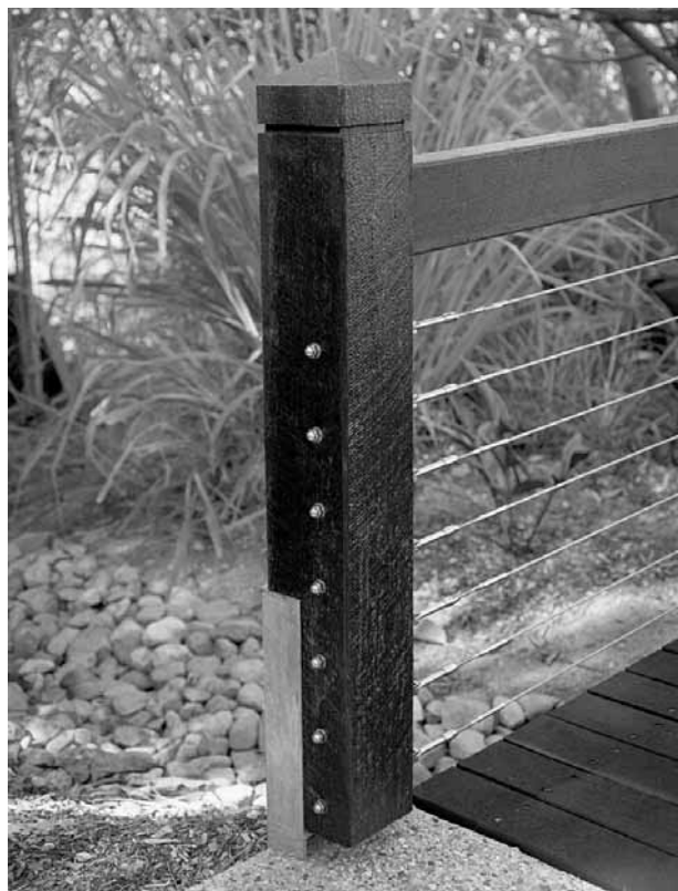
Fig 15 Stainless steel wire as barrier infill.
