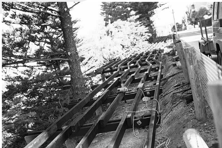
Fig 34 Typical joist framing
