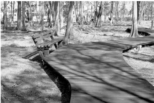
Fig 10 Seat widening
