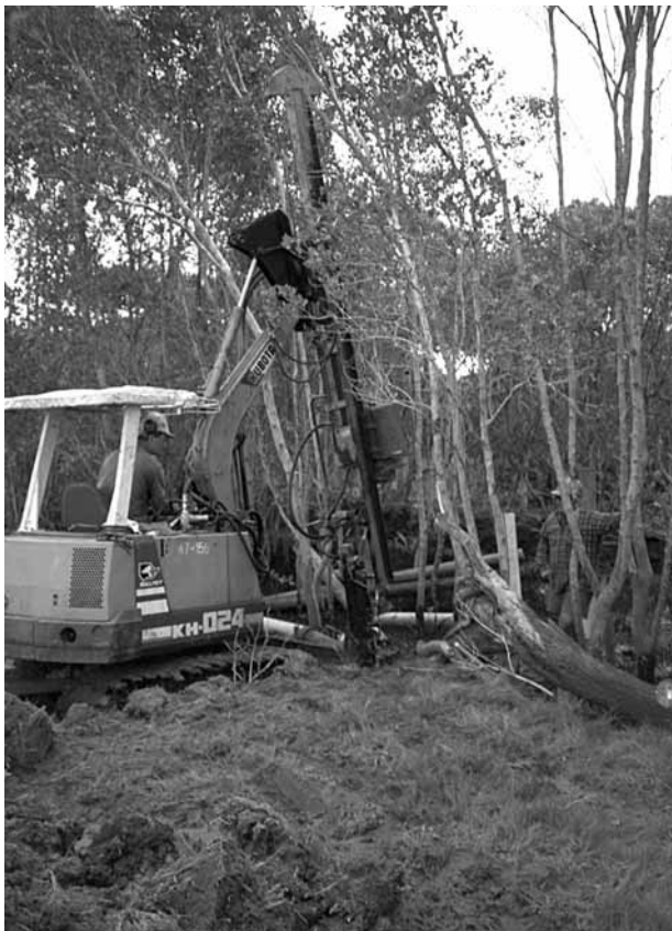
Fig 38 Small pile driver has small footprint
