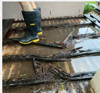
2 year old H3 treated pine deck frame on concrete
