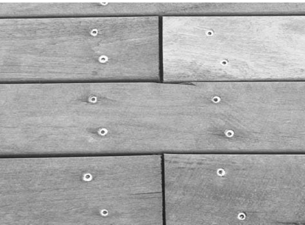
Joining over double joists
