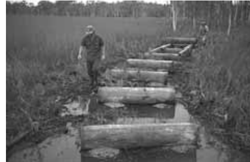
Fig 37 Bedlog installation on poor ground
