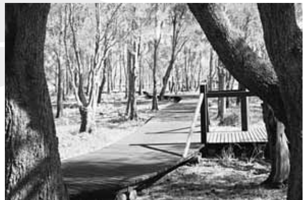
Fig 20 Low boardwalk without edge restraint generally but rails introduced locally to prevent access to fragile marine couch.
