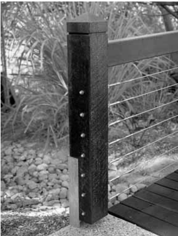
Fig 15 Stainless steel wire as barrier infill.
