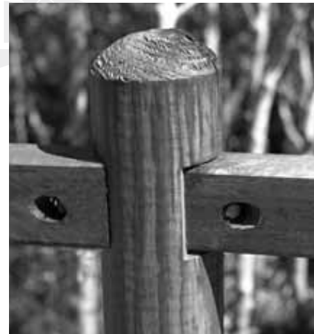
Fig 17 Round handrail post system
