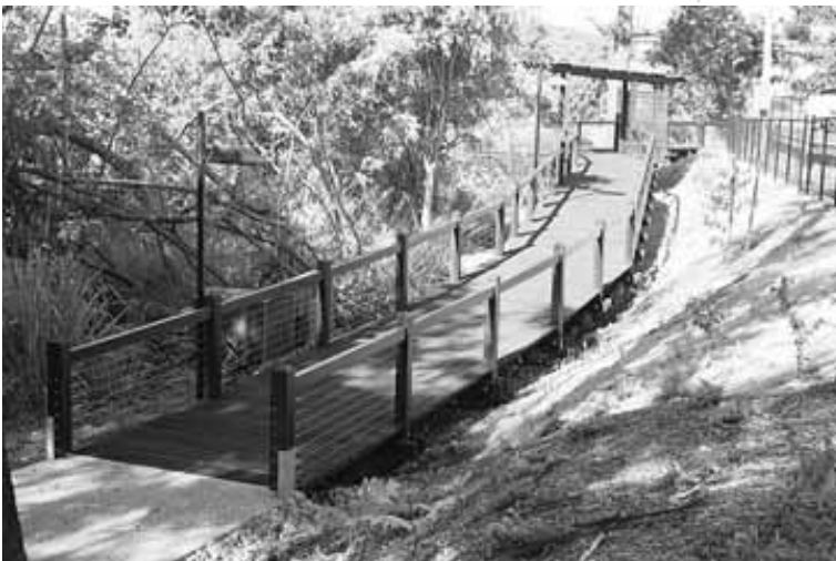
Fig 4. Ramped boardwalk providing access to campus building
