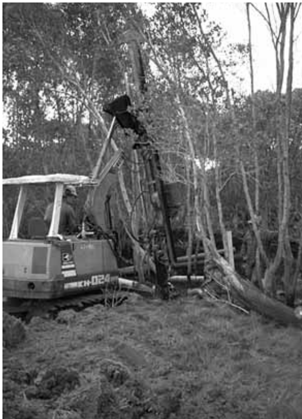
Fig 38 Small pile driver has small footprint
