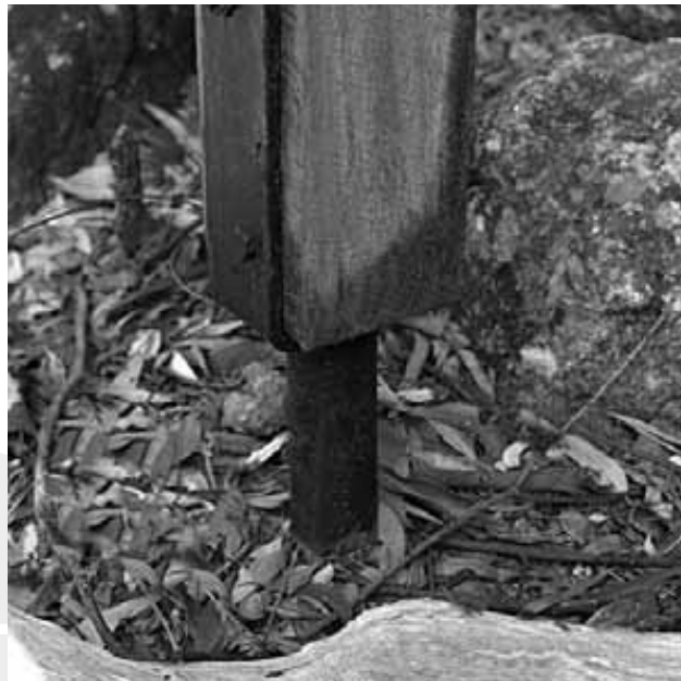
Fig 40 Steel stirrup in cored hole in sound rock
