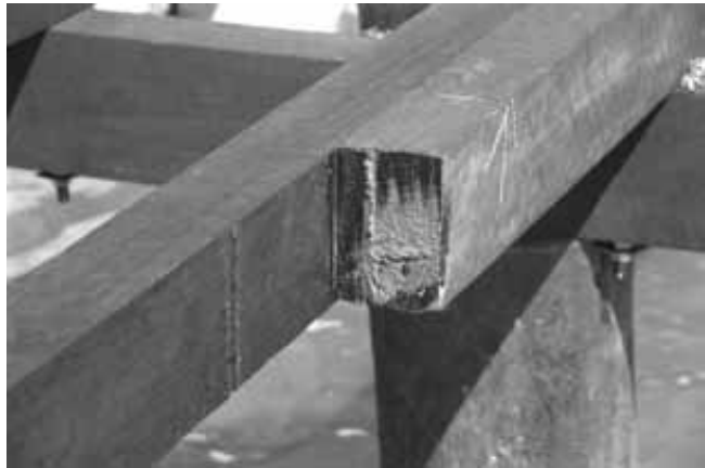
Fig 21 CN Emulsion on cut end
