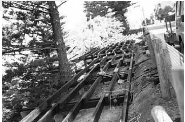
Fig 34 Typical joist framing
