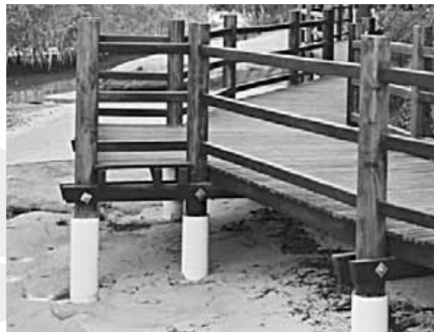
Fig 3 Treated pine piling with UPVC shields in marine environment
