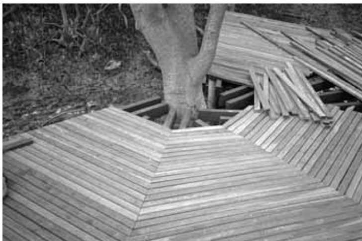
Fig 27 A mitred deck surrounding a specimen tree requires good attention to setting out and experience to achieve a neat result.
