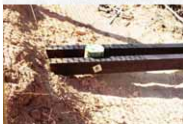
Figure 7 Joists low to ground
