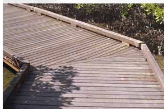
Figure 14 Mitered joint with trimmer
