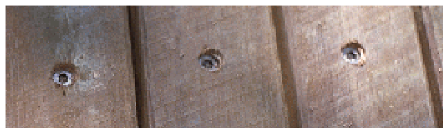
Figure 12 Screws are too deep
