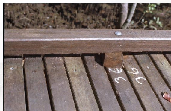
Figure 24 Twisted kerb block
