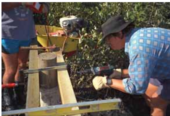
Figure 6 Fitting Headstock
