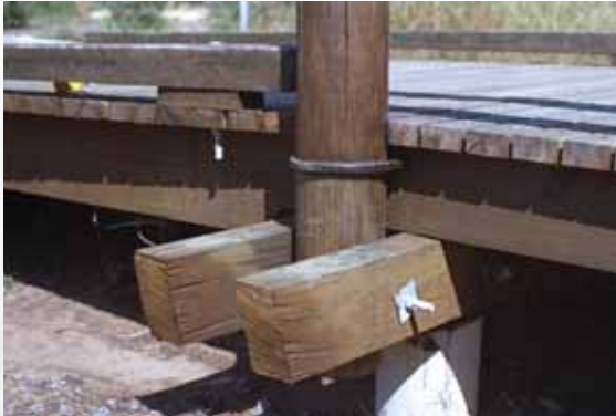
Figure 3 When cut like this, the handrail cannot be braced
