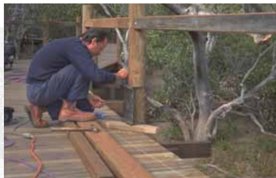
Figure 19 Using a template
