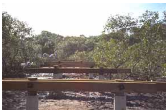
Figure 2 Correctly fitting sleeves through posts cut too short
