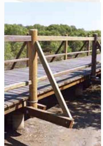
Figure 4 Braced handrail post
