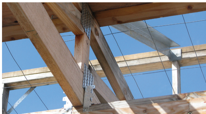
Parapet with HDG steel knee-brace back to main roof
