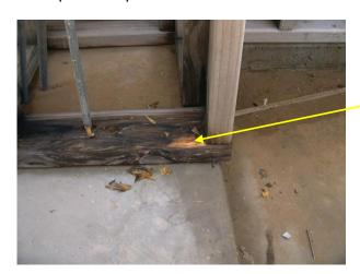
Although heavily discoloured with surface mould and blue stain, the pine timber is still sound as shown by scraping back the surface layer
