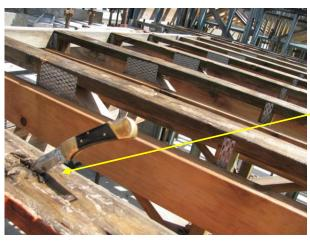
Decayed timber is soft and spongy and can easily be penetrated with a knife or screwdriver
