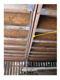
Expansion of the hardwood T&G floor above has caused the separation of double bearers.
